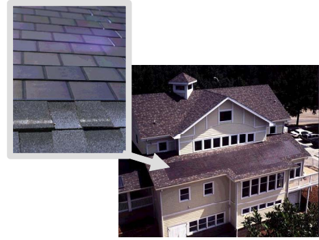
Figure 5 – Example of Amorphous PV Roofing Shingle (Photo credit: NREL)
